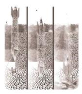
Sandia executed a B61-11 Cable Pull Down stockpile surveillance test at the Sandia Aerial Cable Facility. The test unit was pre-conditioned to the Stockpile-to-Target Sequence cold temperature extreme. Impact conditions were consistent with a low-altitude delivery. Surveillance data were interrogated from the on-board flight recorder, and post-test evaluation indicated the unit functioned normally. NW (1500, 2200, 2900) NW [NW]
